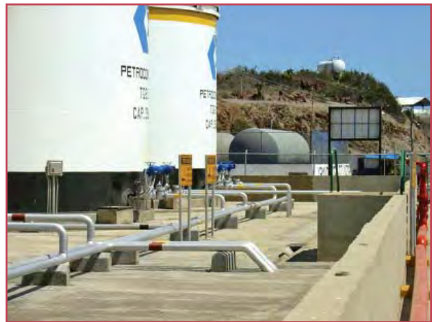
The Baltra fuel handling facility, once an environmental and safety hazard, is now a technologically-advanced facility.
