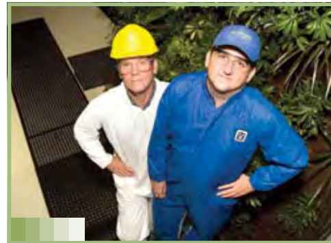
Our plant in Cambridge, Ontario, partnered with the University of Guelph to implement this innovative technology in the paint sludge room: a greenwall that reduces VOCs and odors.
