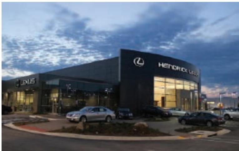
At Hendrick Lexus in Merriam, Kansas, daylight sensors turn off lighting when proper light levels are provided by natural light from skylights and clerestory windows. A programmable lighting control system will automatically turn off facility lighting after hours.
