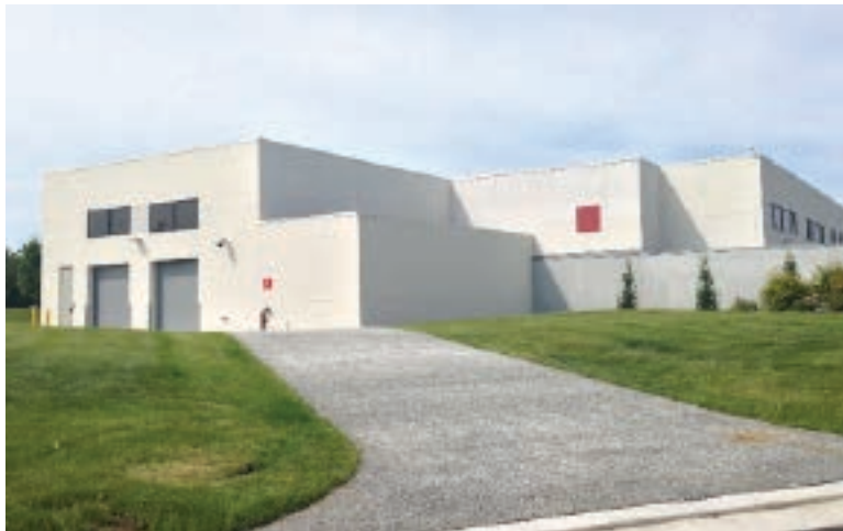
With the expansion of our Technical Training Center in Glen Burnie, Maryland, we are getting a jump on the 2015 launch of our fuel cell vehicle. This center integrates special features to allow for an easy transition to hydrogen vehicle service.
