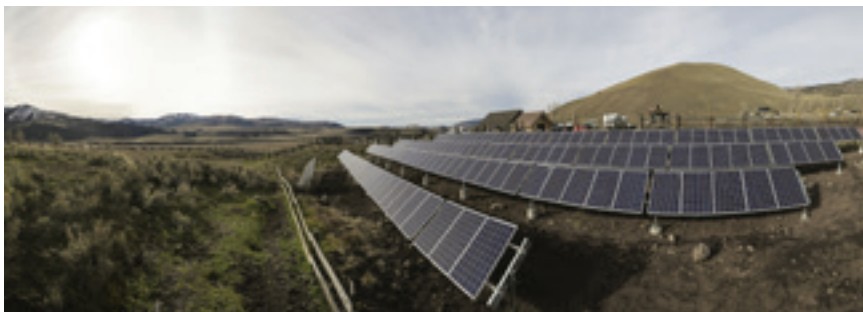
At the Lamar Buffalo Ranch field campus in Yellowstone National Park, 208 reused Toyota Camry Hybrid battery packs (bottom) store energy generated by solar panels (top) in an innovative distributed energy system.
