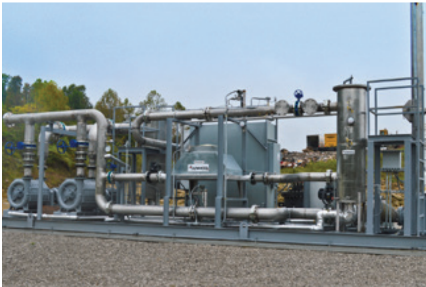
Toyota's plant in Kentucky (TMMK) teamed up with Waste Services of the Bluegrass to generate power from local landfill waste. The blower/flare skid, shown here, is part of the system that extracts gas from the landfill, conditions it and supplies it as fuel to a generator at TMMK. Toyota estimates the landfill gas will supply enough power each year for the production of 10,000 vehicles.
