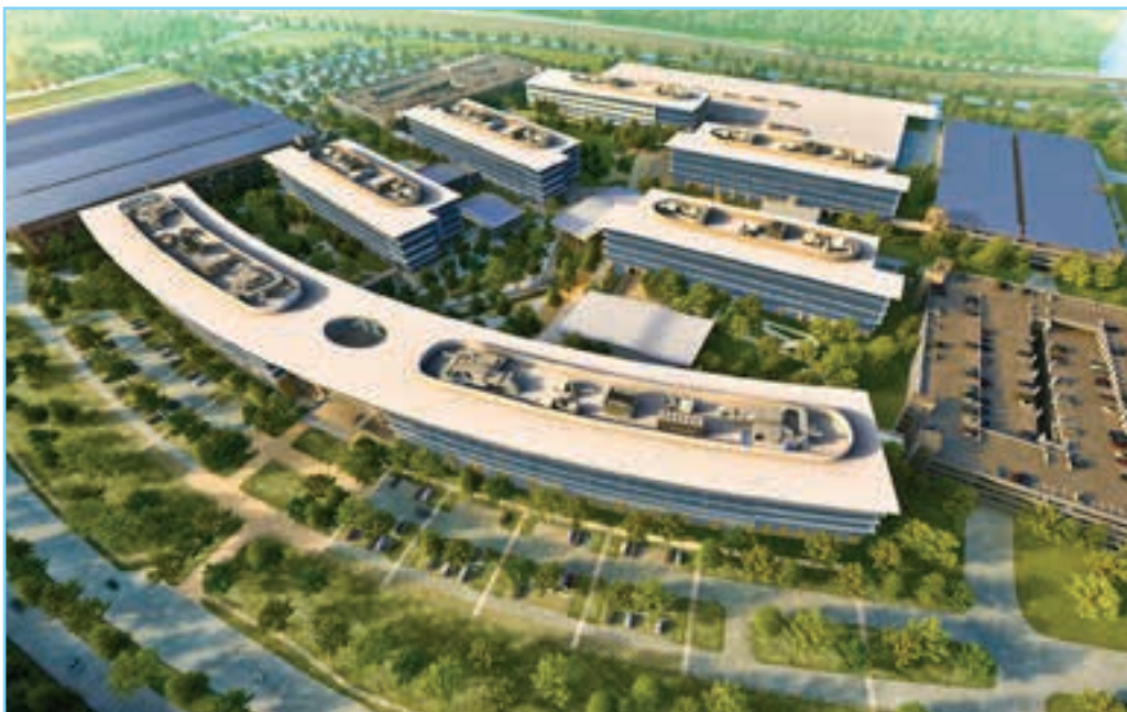
Toyota's new North American headquarters campus in Plano, Texas, will be powered by a 7.75 megawatt solar array that will provide an estimated 25 percent of the campus' energy needs. The system will be the largest on-site corporate office solar installation among non-utility companies in the state of Texas. Completion of the Plano campus is expected in early 2017.
